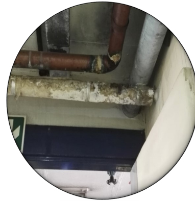
Leaking Pipes
