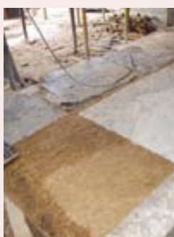
Photo 8. The opening was closed with plywood.
