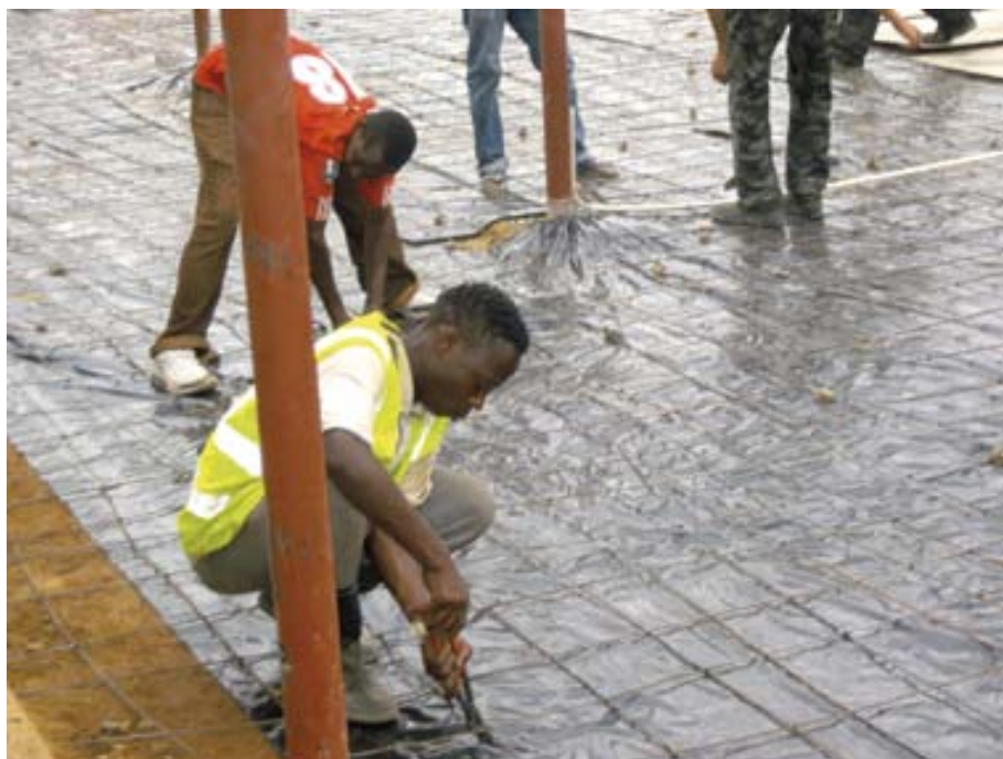
Workers in an awkward posture as they are performing steel fixing work in the preparation to construct a floor.
