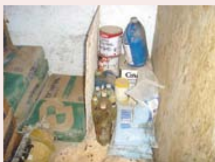
Photo 5. Disorganized storeroom: materials placed in passageway without identification and not separated.
