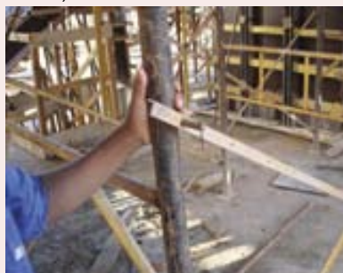
Photo 9. Existence of exposed nails used in the shoring of circulation areas, causing risk of injury to workers.
