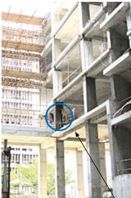
Photo 5. Dangerous working at height. See Training Package: ILO Construction OSH (reference 3)
