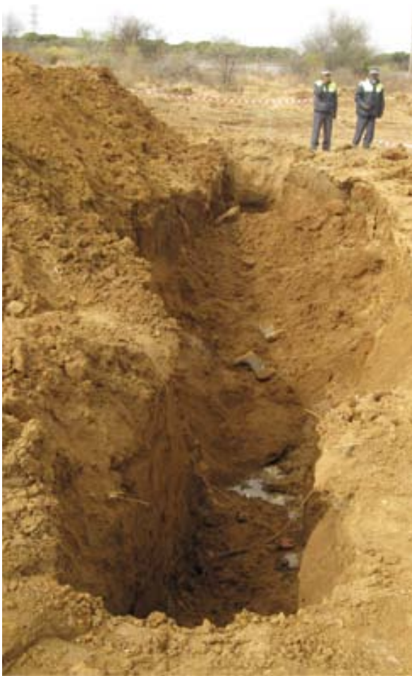
Photo 1. This picture shows a trench 2 metres deep that did not shatter when the walls caved in, causing two fatalities and one case of serious injury.
