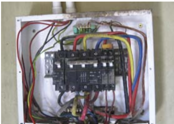
Photo 2. A poorly wired distribution board that caused one death by electrocution.
