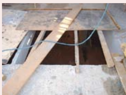
Photo 7. Existence of opening in a floor slab, causing risk of workers and materials falling.
