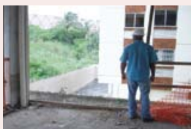
Photo 11. Periphery of slab with no protection, causing risk of workers and materials falling.
