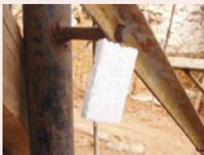
Photo 10. Placing of Styrofoam on all exposed nails.
