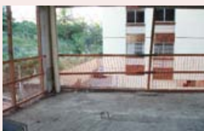
Photo 12. Protection of slab periphery with rails and netting.
